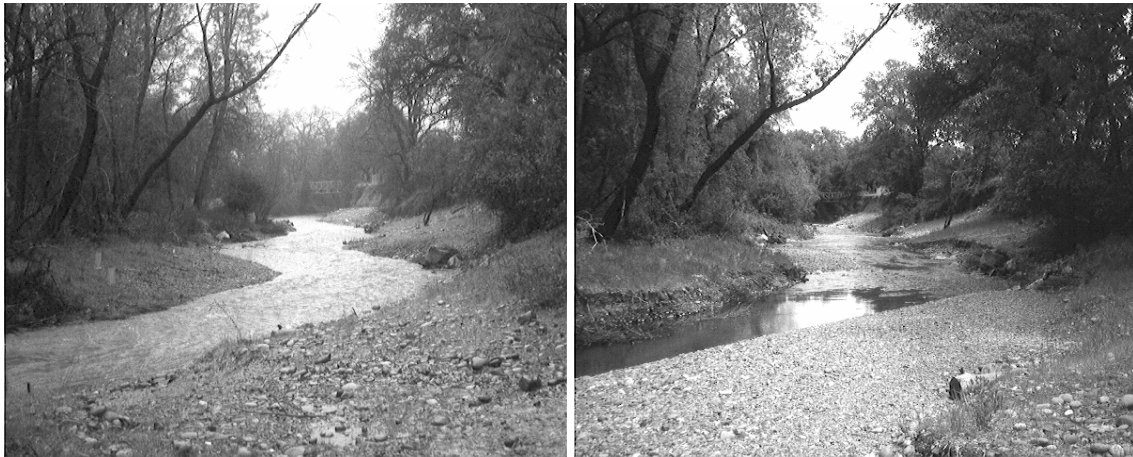
Figure 9 and 10. It is sometimes difficult to envision the dynamic changes that will occur after channel restoration in a seasonal stream, such as the formation of point bars. It is interesting to realize that while the gravels composing the point bars will move through the system, the point bars will still remain. These two photos show the changes that occurred in the new channel after the first large storm event.
