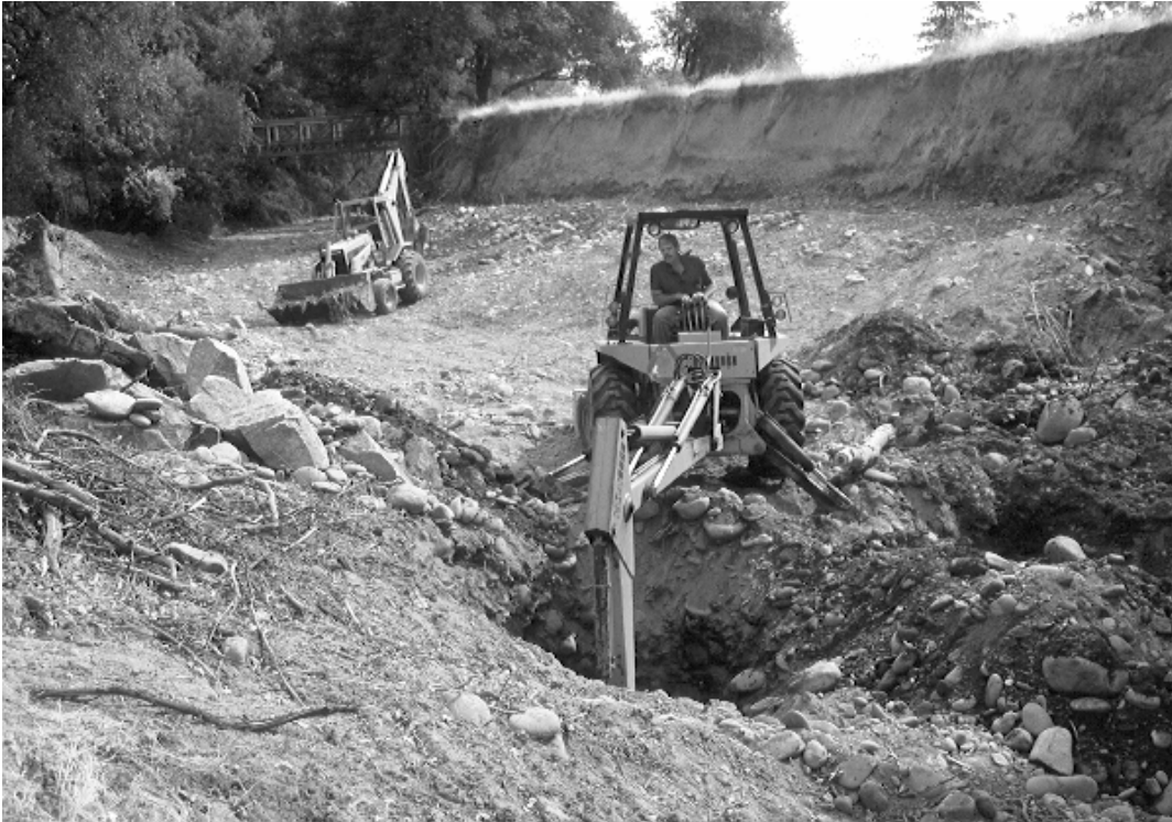
Figure 3. During the channel construction, holes were dug deep in the channel in order to plant the live poles into the vadose zone.
